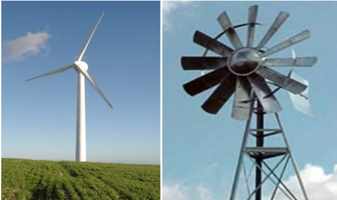
Figure J.5: Eolienne horizontale tripale et multi-pale.
