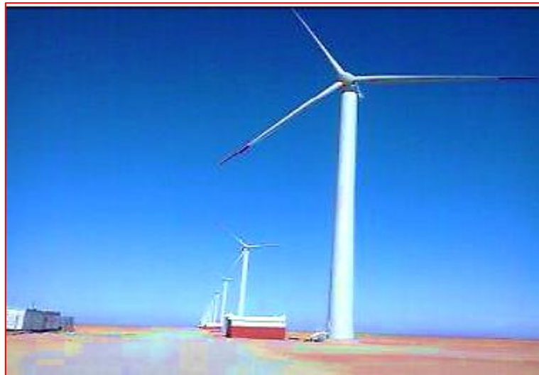
Figure I.3 Adrar wind power plant
