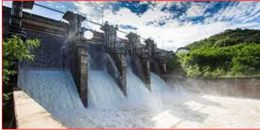
Figure I.5 Dam intended for energy production
