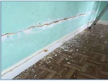
Figure I.9. Fissure horizontale
