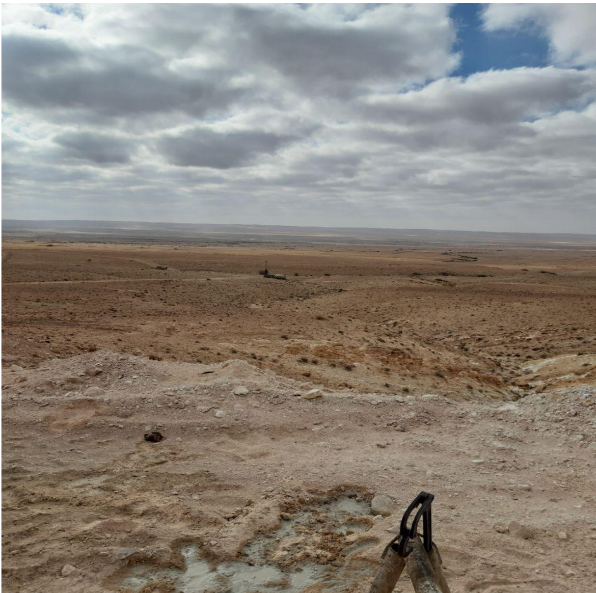
Figure II.6. Chantier de forage.
