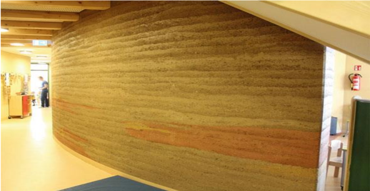
Figure 2.9 Curve shaped (in plan) rammed earth wall (Venkatarama Reddy, 2022)
