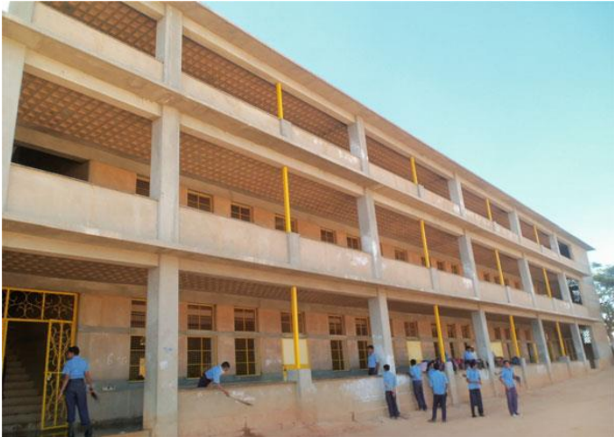
Figure 2.4 Three-storeyed load bearing cement stabilised rammed earth school building, Bangalore, India, built in 2009, corridor has few RC columns for housing rainwater pipes Venkatarama Reddy, 2022
