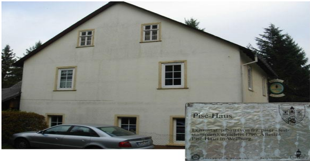
Figure 2.3 Old Pise-Haus (rammed earth house) in Weilburg (Built in 1826, picture taken on 12 October 2008)
