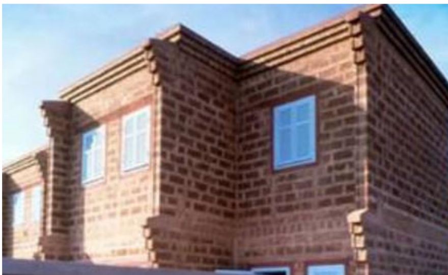
Figure 1.11 Apartments from CEB in Marrakesh, Morocco, ( El Nabouch, 2017) (Guillaud, 1987)
