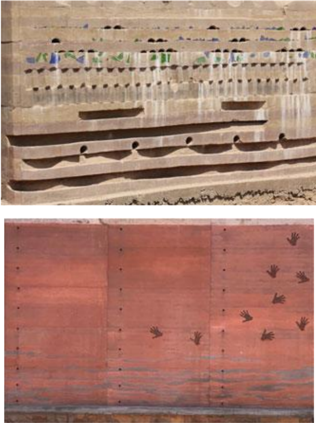
Figure 2.10 Artwork in cement stabilised rammed earth walls at Hunnarashala Bhuj, India (Venkatarama Reddy, 2022)
