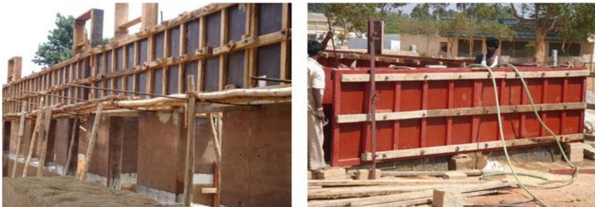
Figure 2.13 Long continuous wooden formwork (Venkatarama Reddy, 2022)
