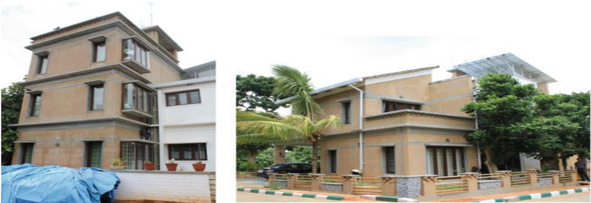
Figure2.5 Three-storeyed load bearing cement stabilised rammed earth residential building, Bangalore, India, built in 2017, designed by architect Mr. Harsha S (Venkatarama Reddy, 2022)
