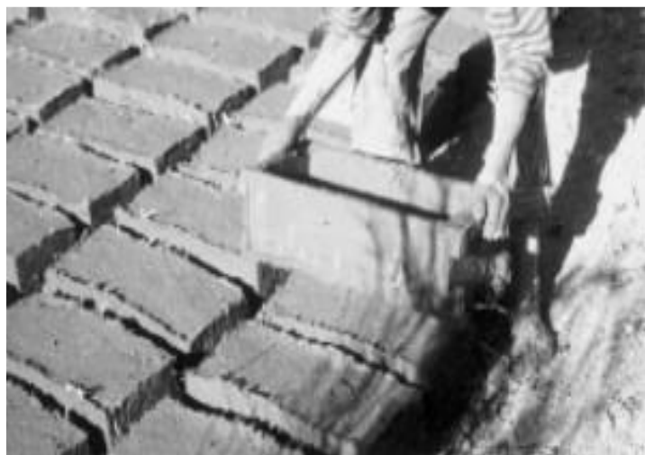
Figure 1.7 Production of Adobe in Ecuador, (El Nabouch, 2017) (Minke, 2001)
