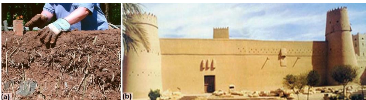
Figure 1.9 (a) Technique of Cob construction; (b) Masmak Castle in Riyadh, Saudi Arabia (El Nabouch, 2017)
