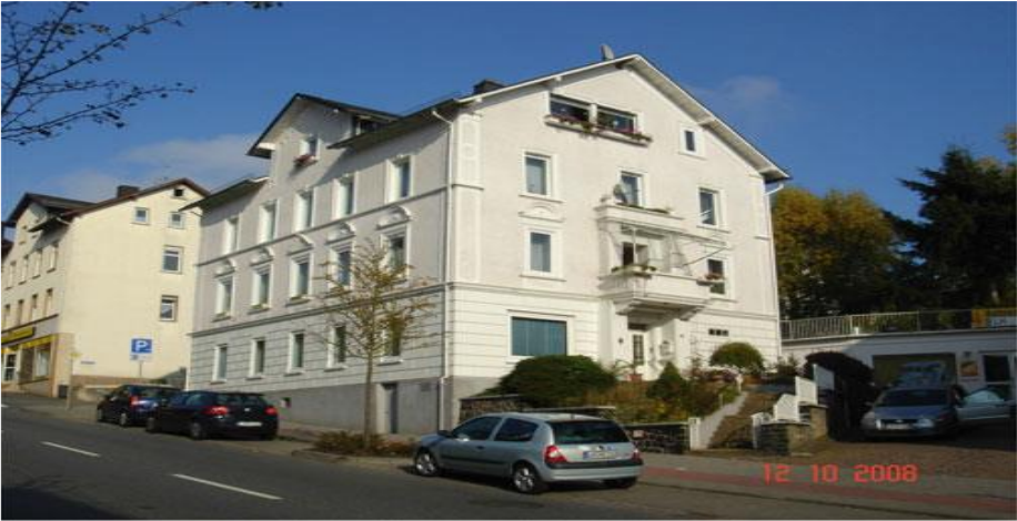
Figure 2.1 Unstabilised rammed earth house, Weilburg, Germany, (Constructed in 1850, picture on 12 October 2008 (Venkatarama Reddy, 2022)
