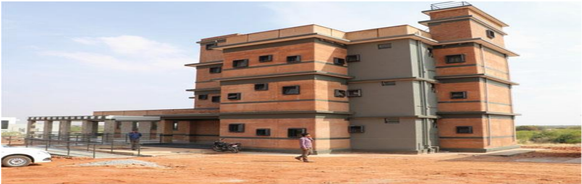
Figure 2.6 Three-storeyed load bearing cement stabilised rammed earth dormitory building, India, built in 2019 (Venkatarama Reddy, 2022)
