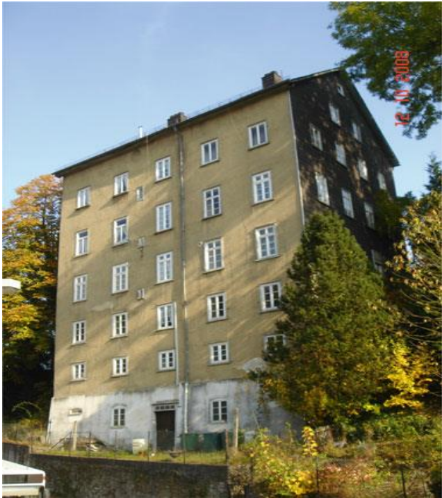
Figure 2.2 Sixstorey load bearing unstabilised rammed earth building, Weilburg, Germany, (Constructed in 1826, picture on 12 October 2008) (Venkatarama Reddy, 2022)
