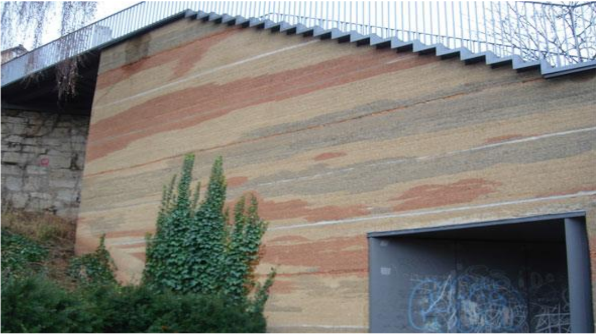
Figure 2.8 Different coloured textures in rammed earth using natural soils (Venkatarama Reddy, 2022)
