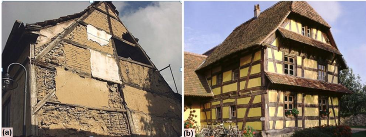
Figure 1.6 (a) Building in the central German city of Bad Langensalza made of wattle and daub and (b) House in France, Alsace (El Nabouch, 2017)
