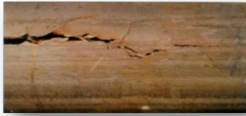
Figure I. 6: La corrosion sous contrainte
