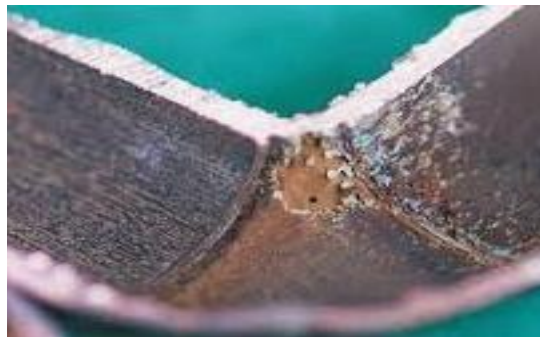
Figure I.10: La corrosion sous contrainte
