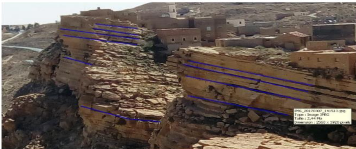
Figure33: photo illustrant les joints de stratification.
