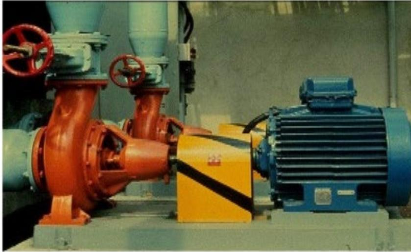
Figure IV . 2 Pompes centrifuge
