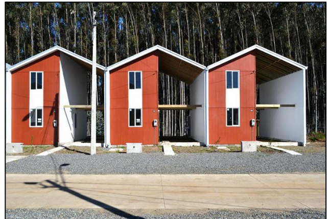
Figure 56: Half a house de Villa Verde, Chili. Source : archdaily.com
