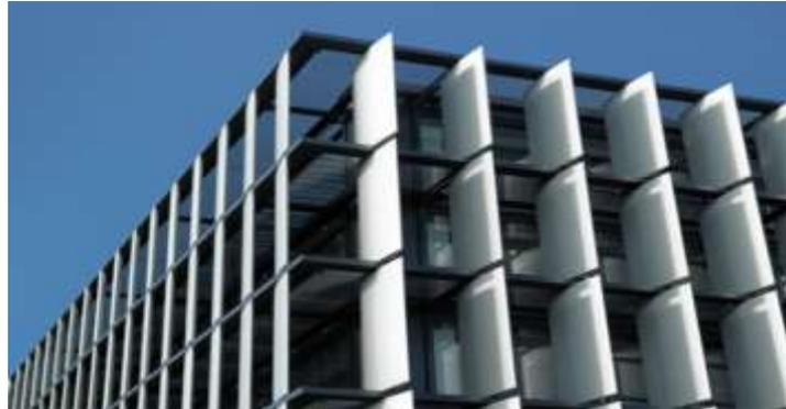
Fig3.4 solarfin qolt France (panneau) Source :( revu integred building 2021)
