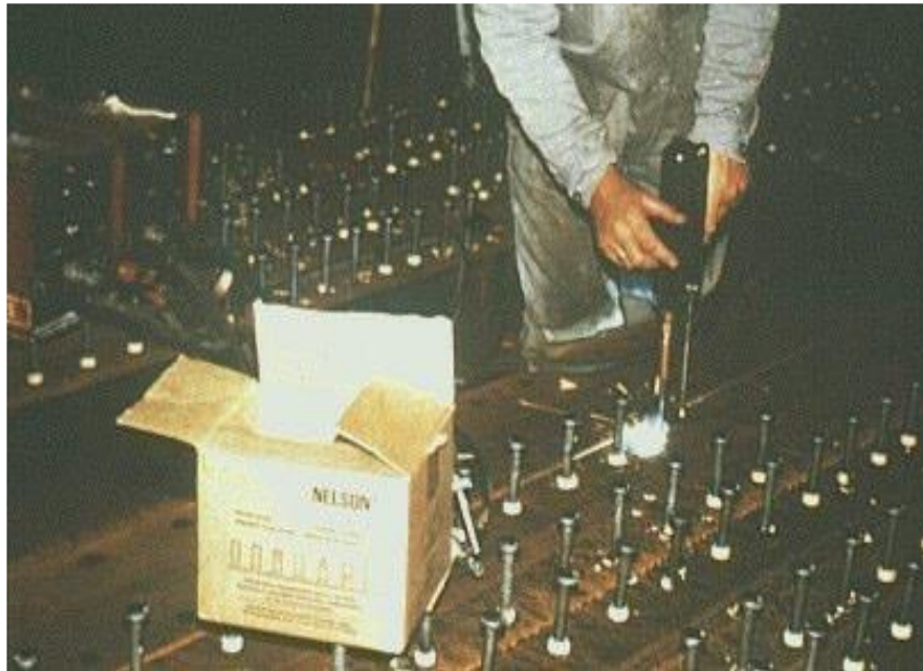
Figure 1.7 Welding the Shear Studs to the Steel Flange
