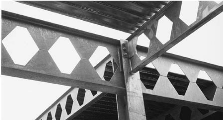
Figure 1.3: Example of castellated beams
