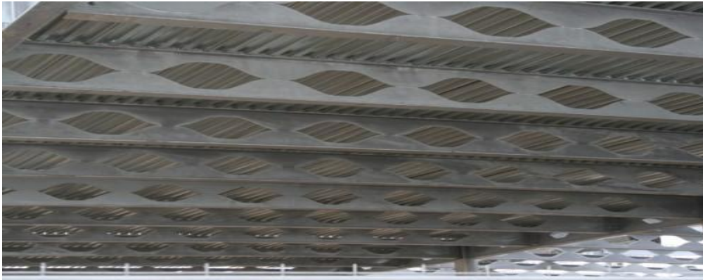
Figure 1.9: Angelina beams
