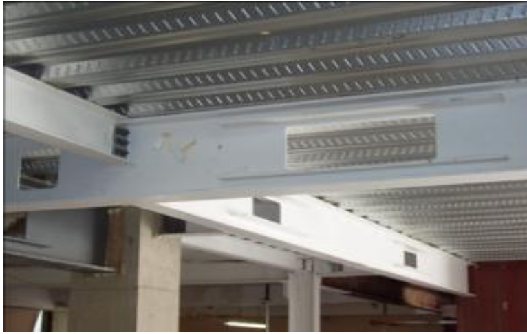
Figure 1.7: rectangular shape with large reinforcement
