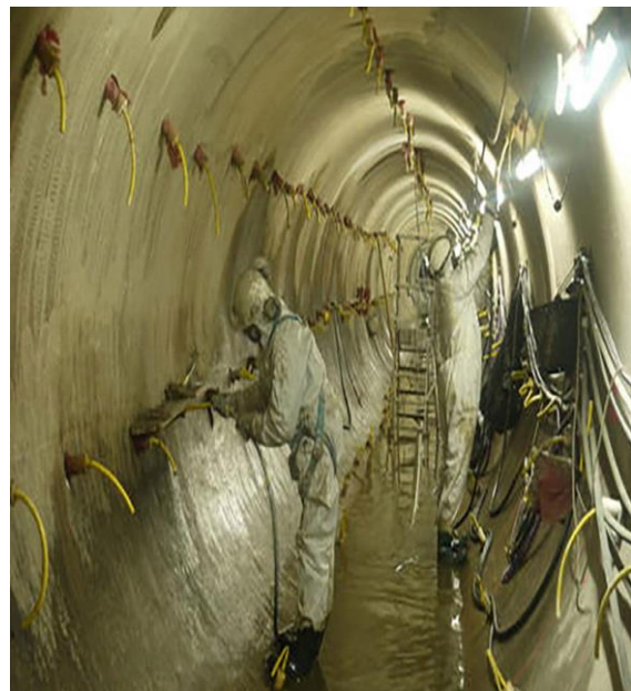
Figure I. 16. Injection de consolidation [5]
