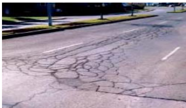
Figure II. 15. Faiénçage
