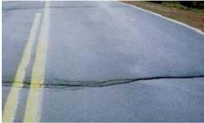
Figure II. 12. Fissures transversals
