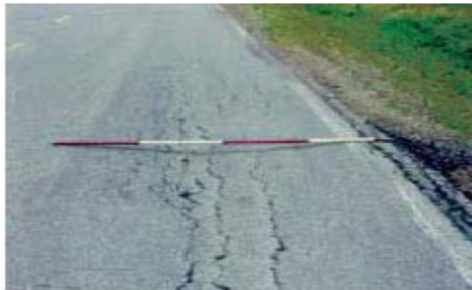
Figure II. 11. Affaissements
