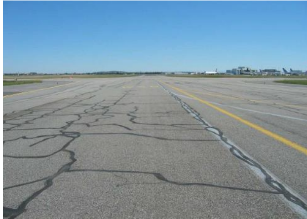
Figure II. 14. Fissures anarchiques
