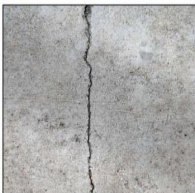
Figure 1.8 fissure verticale [9]
