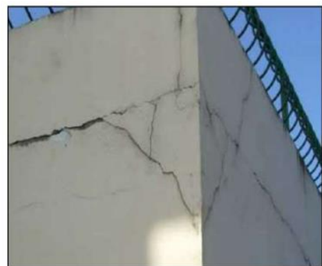
Figure 1.9 les microfissures [8]
