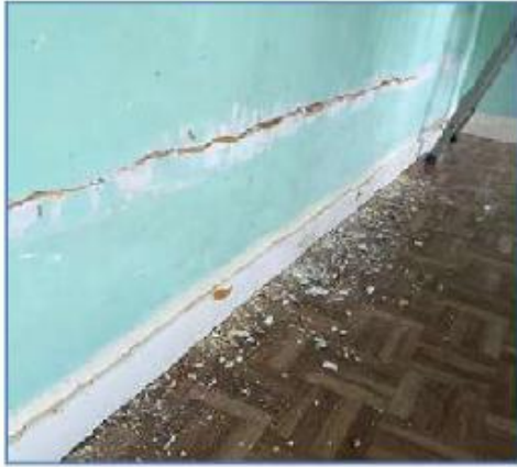
Figure 1.10 : fissure horizontale [8]
