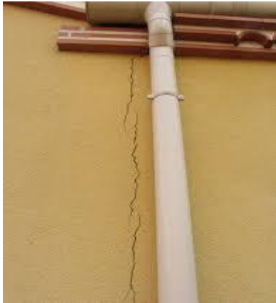
Figure 1.7 fissure verticale.
