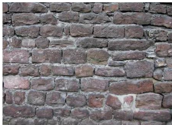
Figure 2-3 Stone Masonry Construction
