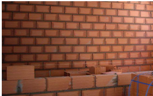
Figure 2-1 Brick Masonry Construction
