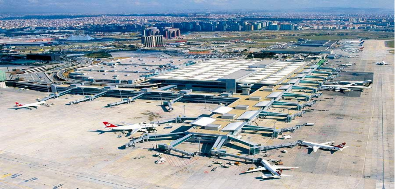
Fig 3.4: Parking areas of ATATURK airport (Turkey). [26]
