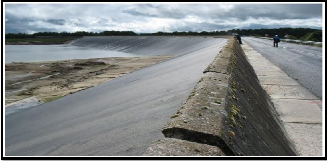
Photo II.08: barrage de Monne (CFBR, 2012)
