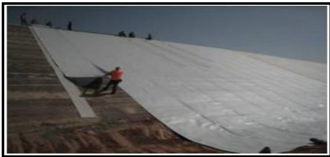
Photo II.09: Pose de géomembrane (barrage de Sar Cheshmeh, Iran)
