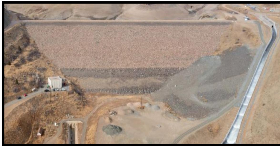
Photo III.04: protection du parement aval (USBR, 2012)
