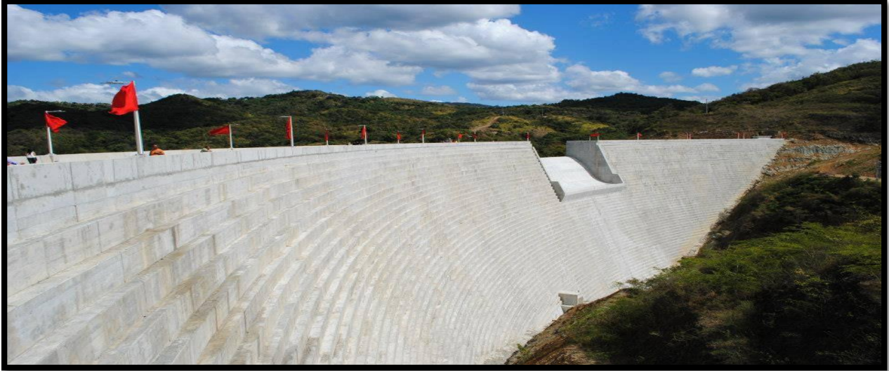
Photo IV.04: barrage portugues, porto rico (US army corps of engineers, 2014)
