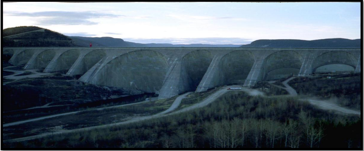
Photo I.06: barrage Daniel Johnson 214m, Quebec (JM Chouinard)
