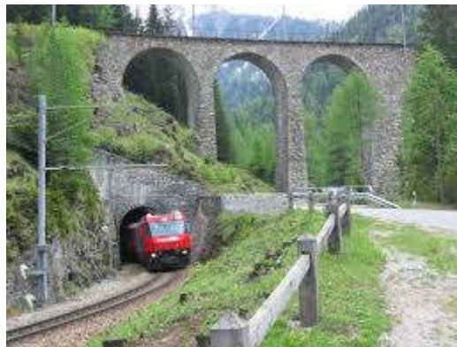
Figure III.1 Tunnel en spirale.
