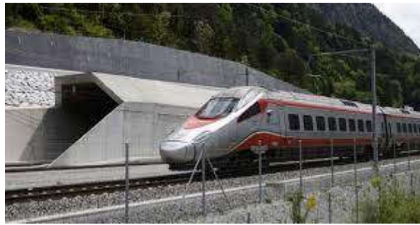
Figure III.2 Tunnel hors embranchement.
