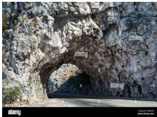
Figure III.13 Tunnel en roche dure.
