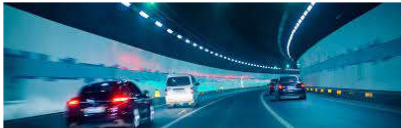
Figure III.6 Tunnel de circulation.
