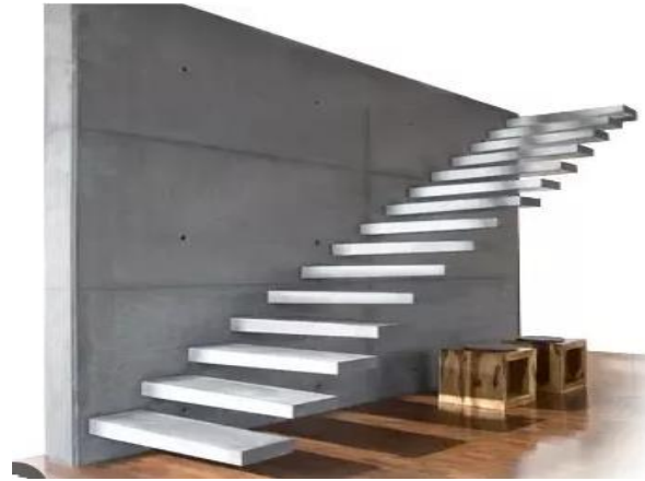
Figure 1.10: Example of application of cantilever beam
