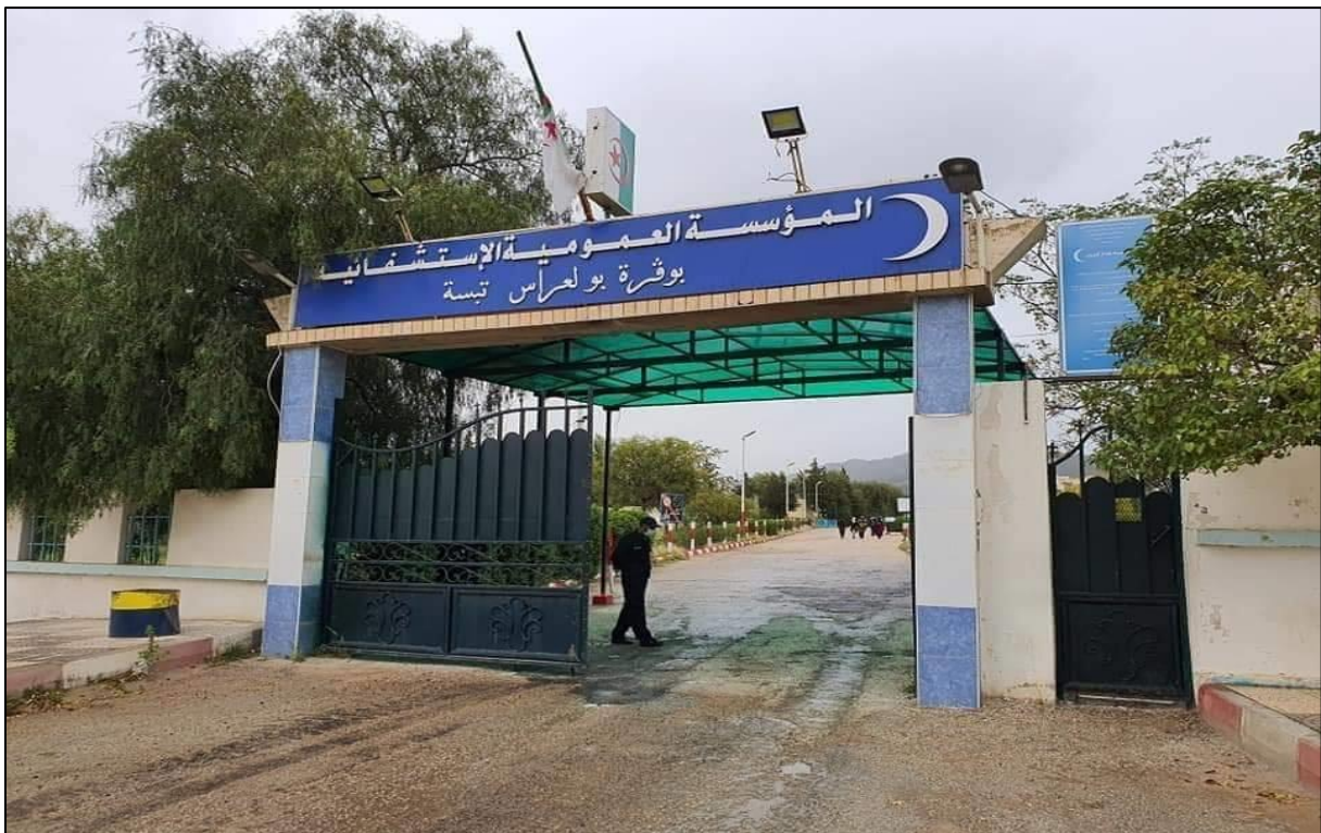
Figure 33: l'Etablissement public hospitalière (Bouguerra Boularès Bekkaria)
