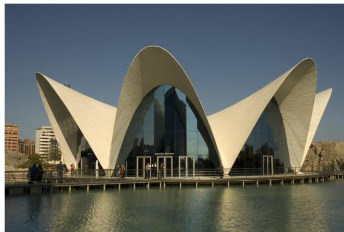
Figure 1. 14 Thin shell FRC structure in Valencia, Spain
