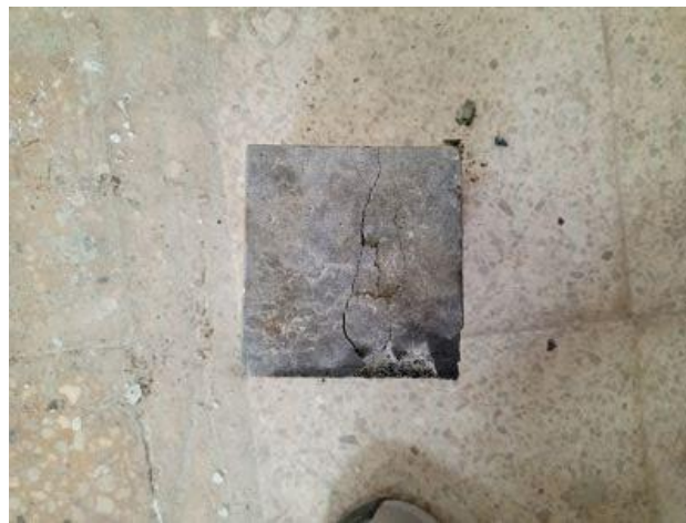
Figure 3. 5 enhanced structural integrity of concrete compared to previous specimens
