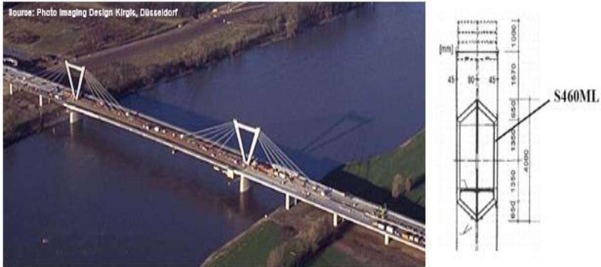
Figure2. 12Rhine bridge Düsseldorf-Ilverich with tension tie in the pylons made of S460 TM
