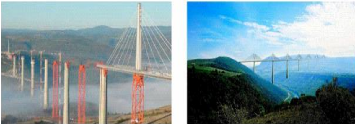
Figure2. 13Millau-Viaduct and launching of pylon
