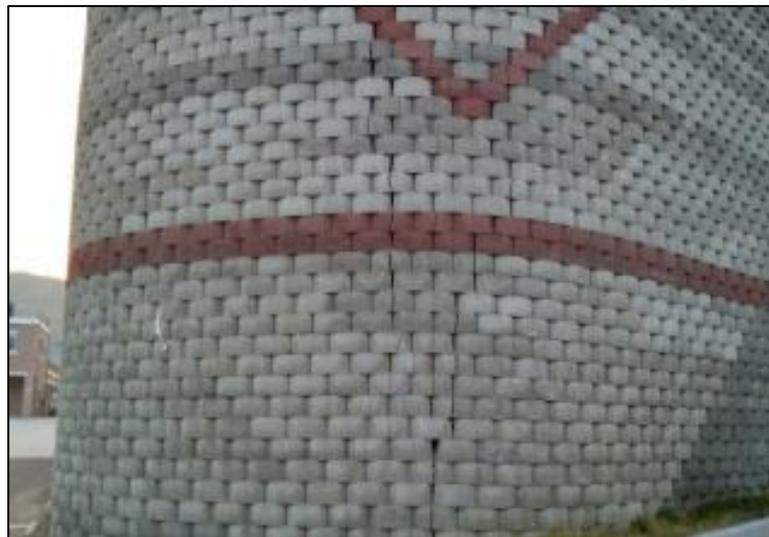
*Figure3.3. Fissure et bousculade (Korean Geosynthetics Society, 2010)*
