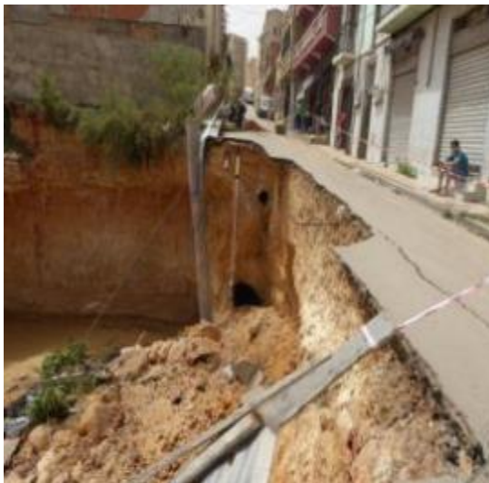
(c) Mila (Type: Deep-Rotational landslide; Date: September 2013)
