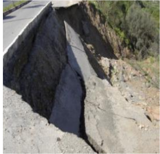
(b) Sibari (Type: Shallow-Planar landslide; Date: February 2008)
