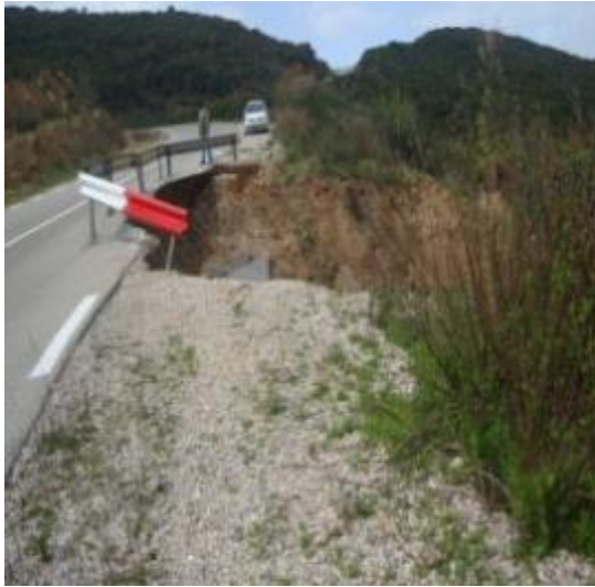
(a) RN 79a, (Type: Deep-Rotational landslide; Date: October 2011)
