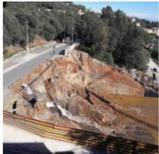
(d) Grarem (Type: Planar landslide; Date: June 2015)
