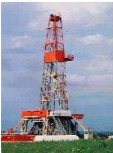
Figure II.07. Mat de forage [7]
