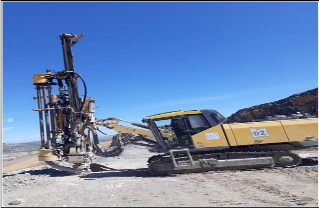
Figure V.9. Foration verticale des trous
