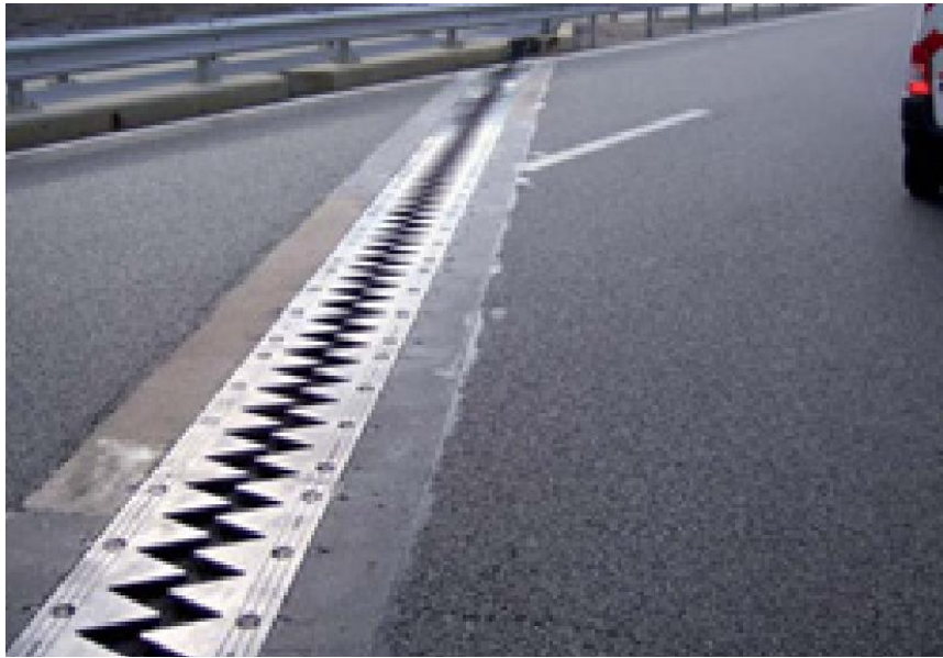
Figure 14. Joint de dilatation [9].
