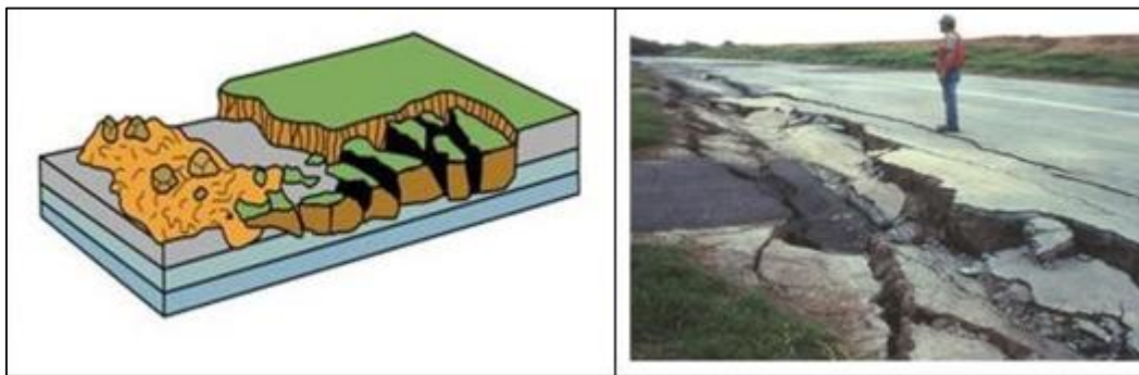
Figure I.16: Schematic view and photo of spread in California, USA in 1989 (Highland et al, 2008)
