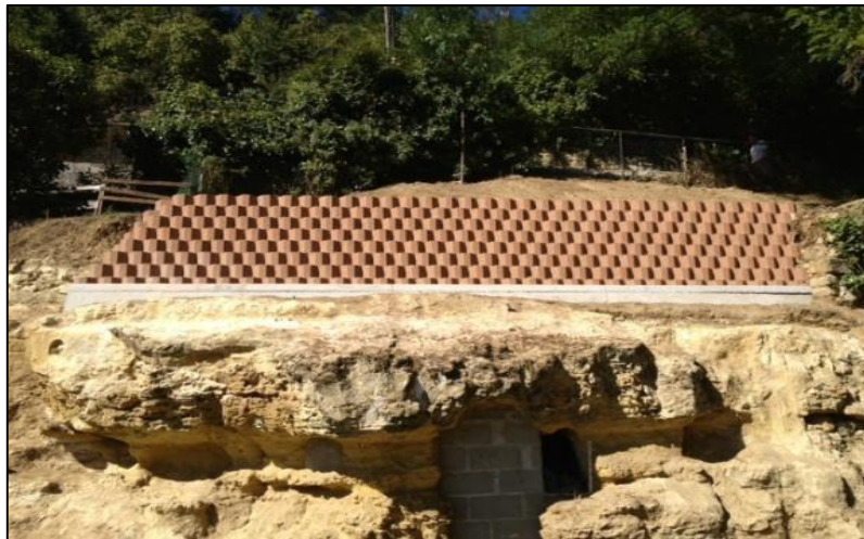
Figure I.32: Retaining wall in Chinon, Image Pinon SA.
