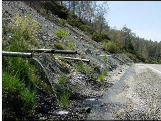
Figure I.29: Slope drainage by barbicanes, image (University of Illinois at Urbana-Champaign, Department of Geology)
