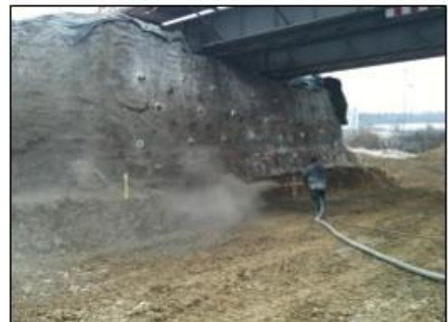
Figure I.30. Nailing principle and example of realization, SIMPRO image
