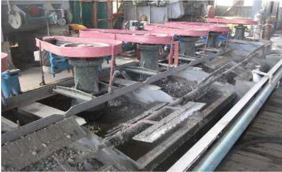
Figure I.18 : Cellule de flottation type Denver.
