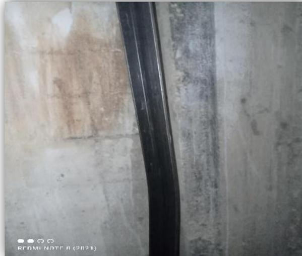
**Figure IV.28.** Rail de guidage.
