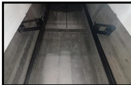
**Figure IV .7.** Deux rails de guidage.
