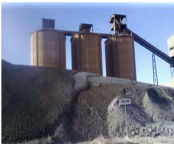
Figure II.26. Silos de stockage du clinker.
