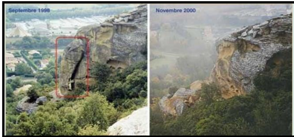
Figure 32 : Rupture de pied (guide technique, 2004)
