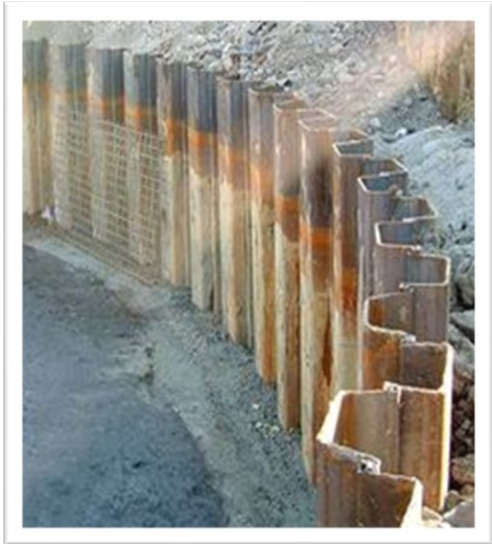
Figure 4: backfill stabilized with sheet piles
