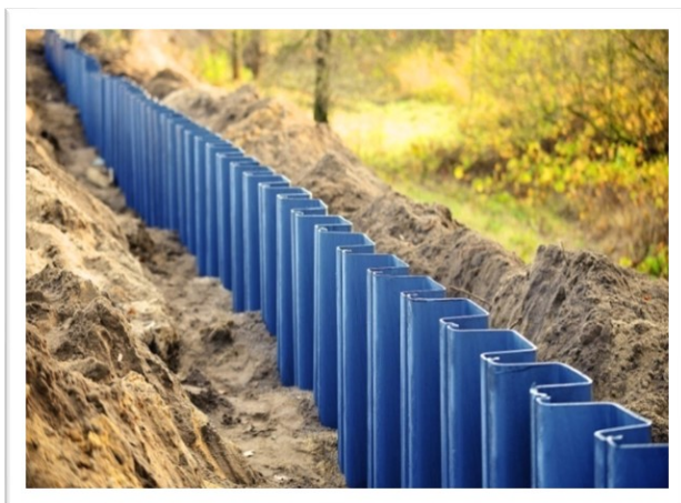
Figure 1: Sheet piles assembling
