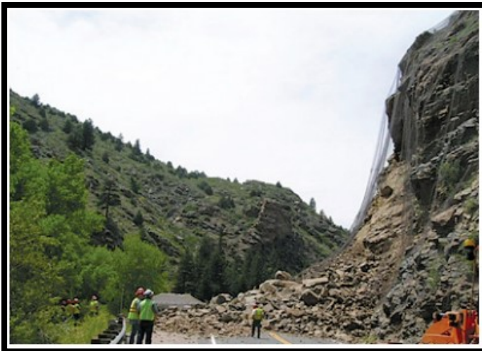
Figure 3: A rock fall/slide that occurred in Clear Creek Canyon, Colorado, USA,
