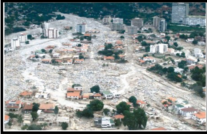
Figure 13: Debris-flow damage to the city of Caraballeda
