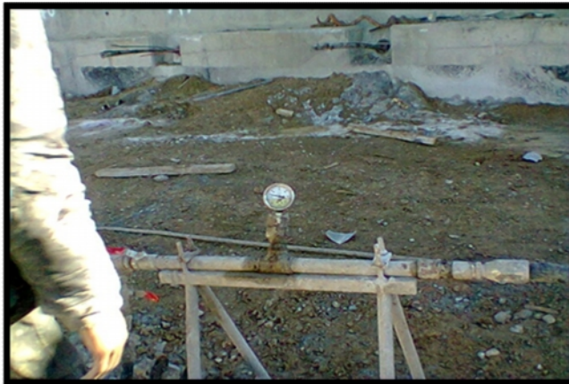
Figure 3 .7 L'injection de coulis
