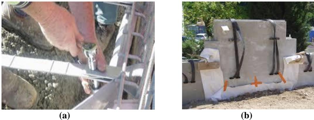
**Figure 2.11** : Connexion Parement/Armature
