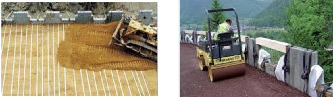
**Figure 2.15 :** Remblayage et compactage [7]
