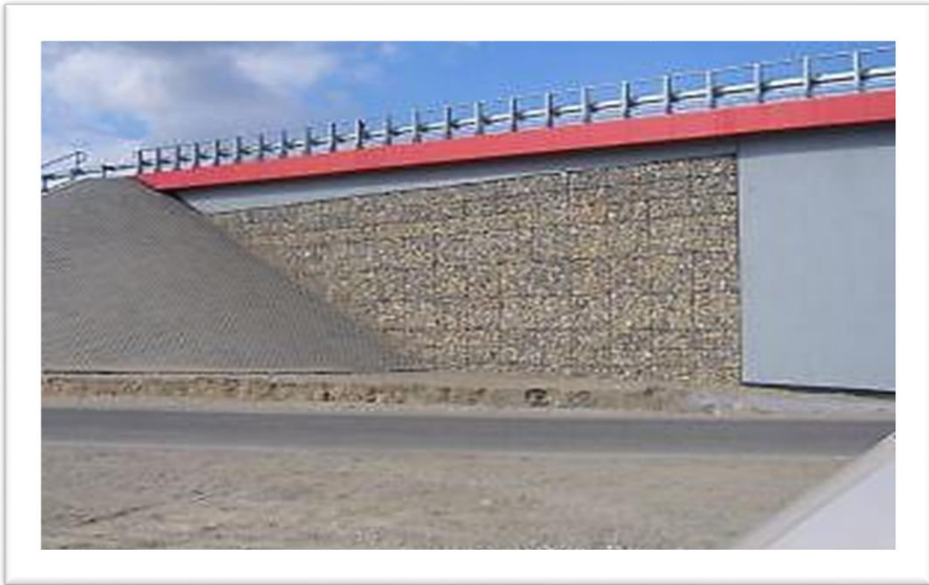
Figure 2.13 Mur de gabion [36]
