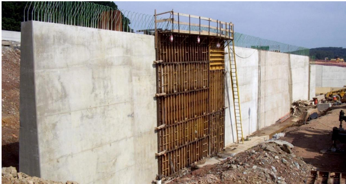
Figure 1.21 Reinforced concrete retaining wall
