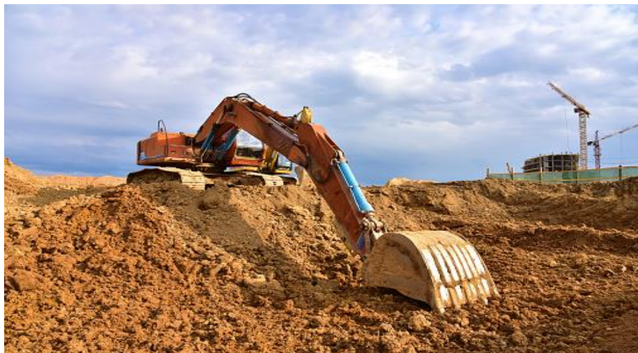
Figure 1.7 digging a pit foundation
