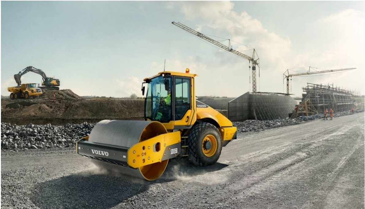
Figure 1.9 Soil compaction for road building
