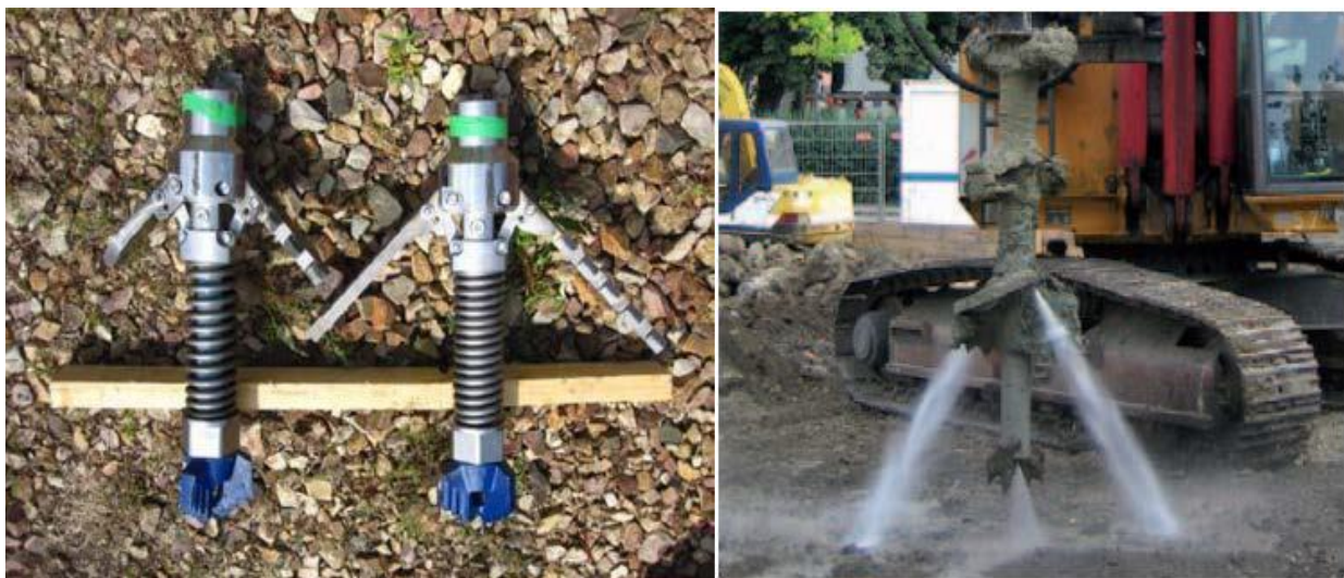
Figure 2.2 Examples of simple rotary tools. Augers used to wet mixing: a) Springsol® by Soletanche Bachy (Guimond-Barrett, et al., 2012), b) DSM rotary tool by Keller (KELLER, 2013)
