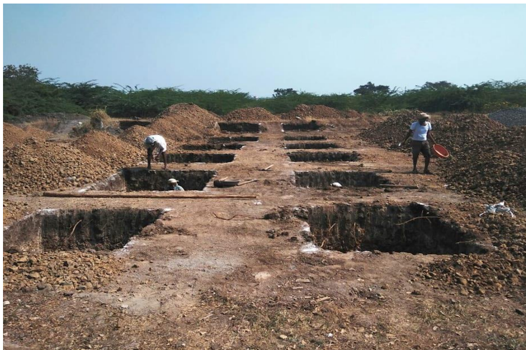
Figure 1.12 Footing excavation
