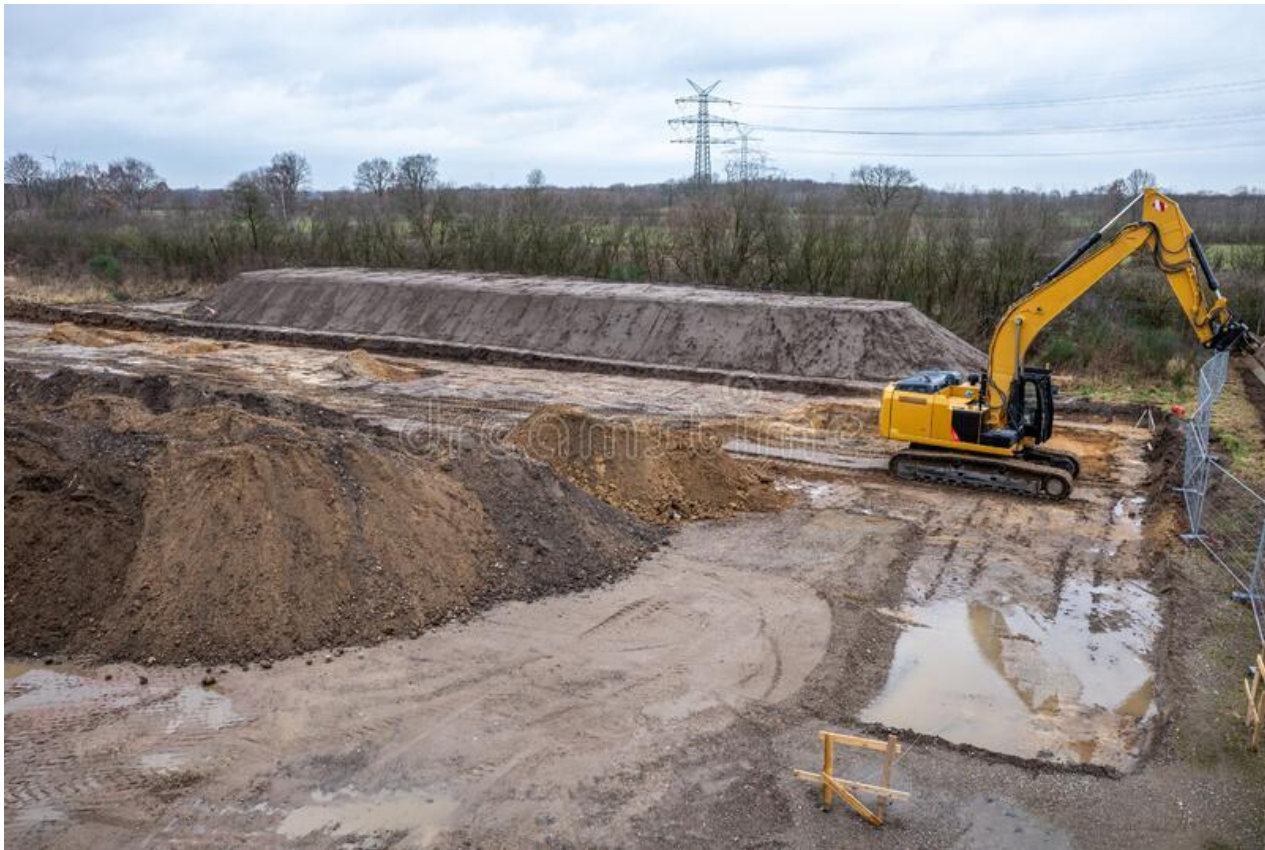
Figure 1.10 Top soil excavation
