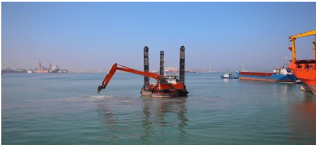
Figure 1.15 Dredging excavations
