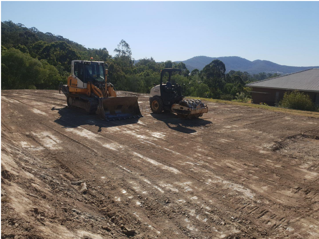
Figure 1.8 Site leveling and compacting
