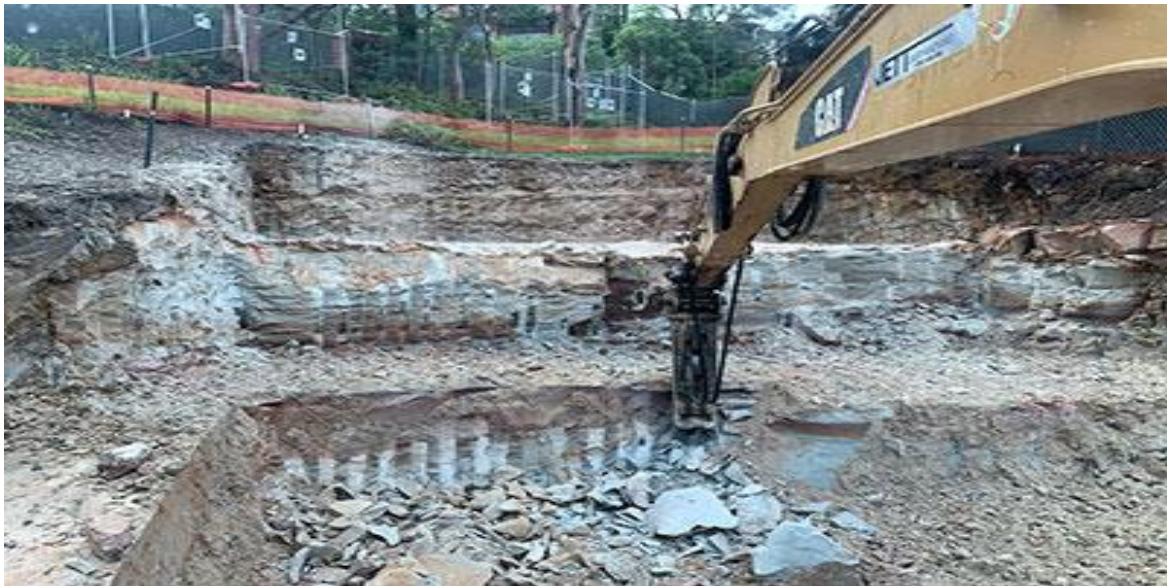
Figure 1.11 rock excavation
