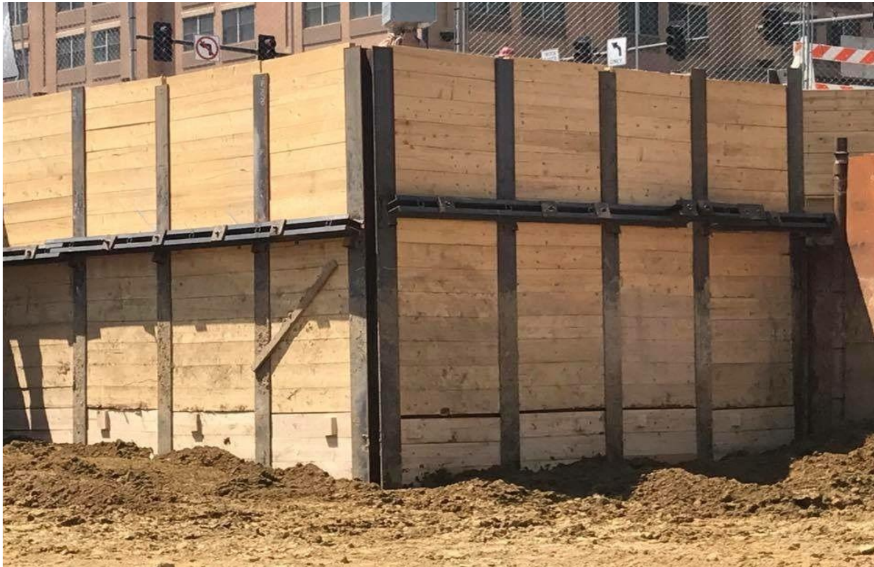
Figure 1.16 soldier pile wall and laggings
