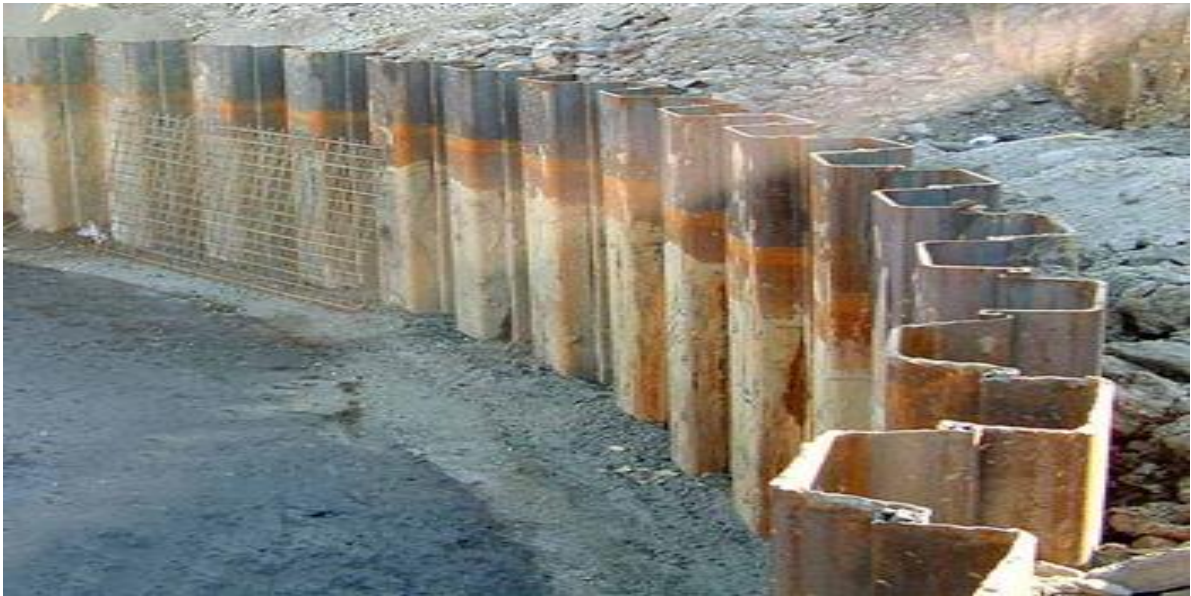
Figure 1.18 sheet pile wall
