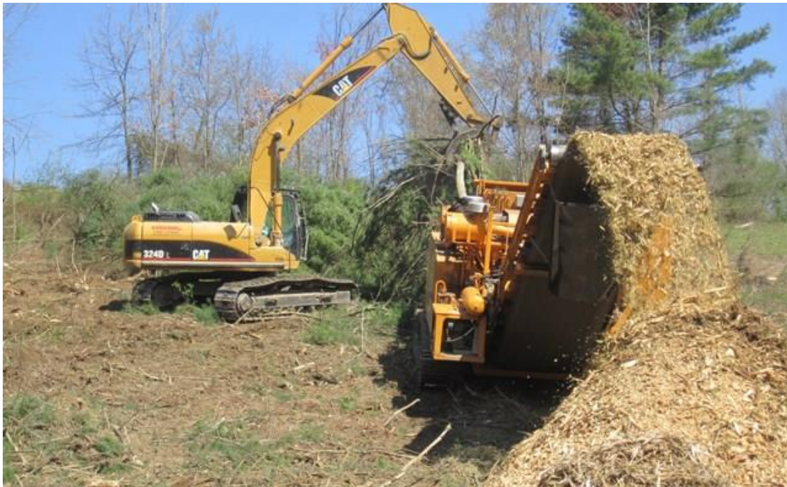
Figure 1.4 Land clearing and grubbing
