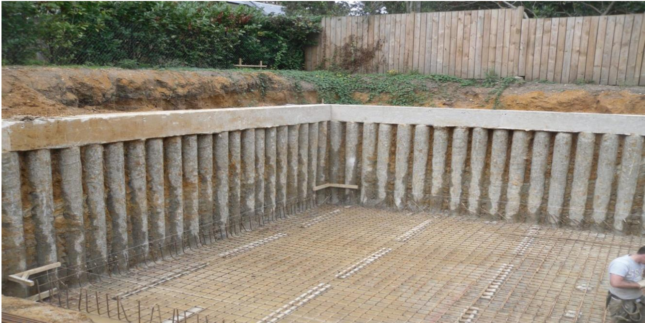
Figure 1.19 Pile wall
