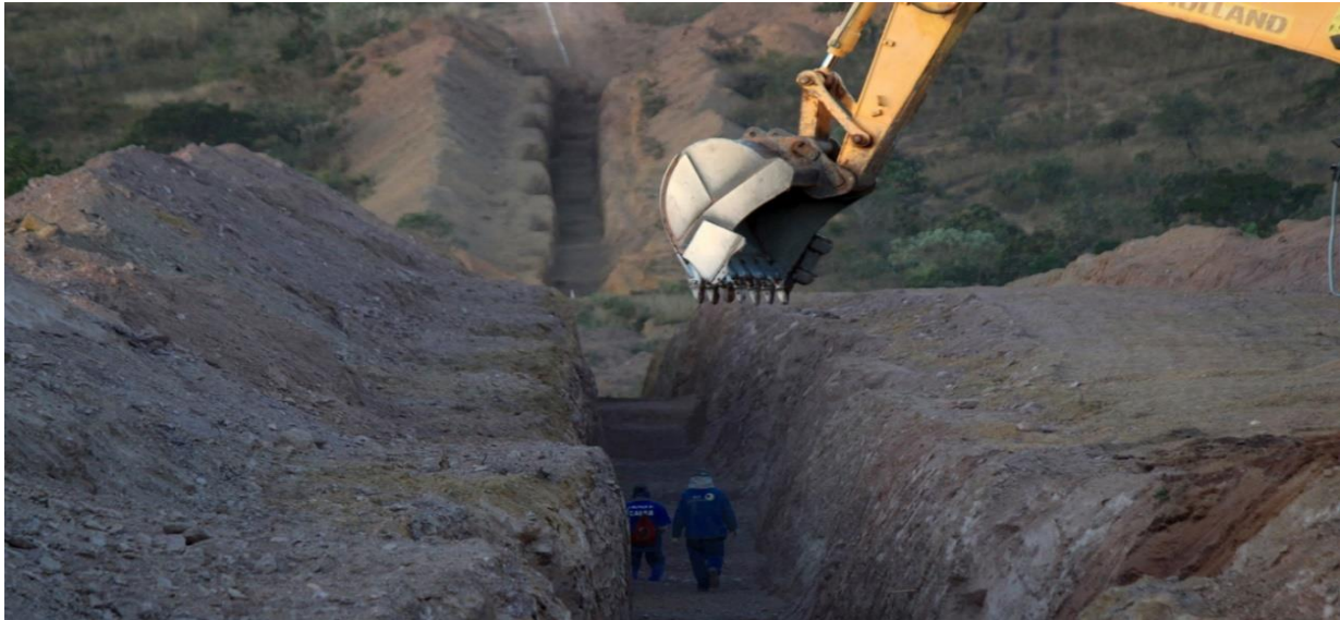
Figure 1.14 Trench excavation
