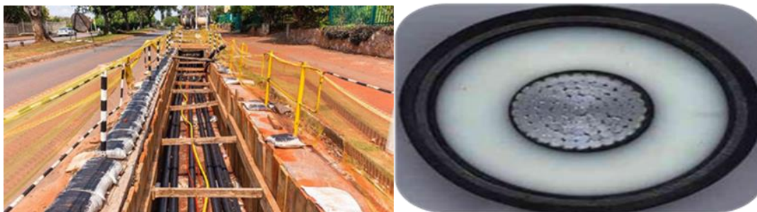
Figure.1.2. Câble HTA souterrain.
