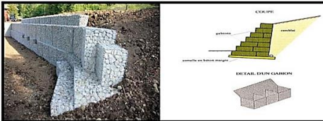
Figure 1.2 Murs de gabions.
