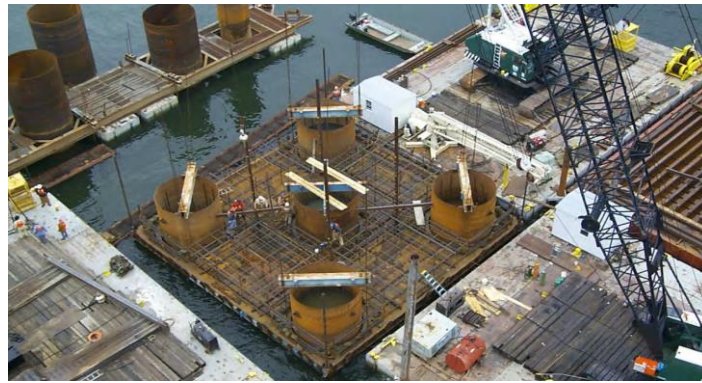
Figure 3.8 Group of Drilled Shafts for Large Loads
