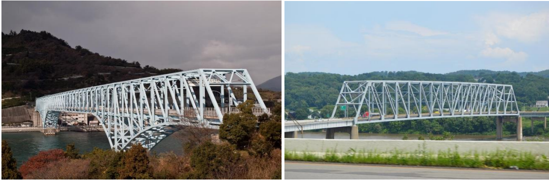
Jennings Randolph Bridge (WV, USA)
