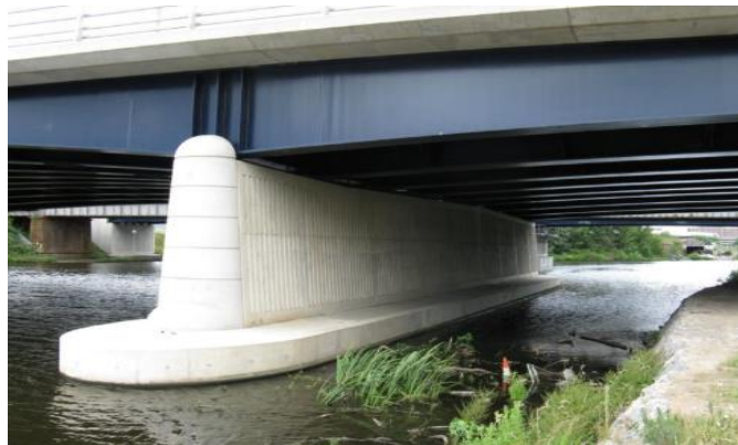
Figure 2.5 Solid Reinforced Concrete Piers
