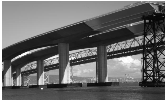
Figure 2.2 Columns in Skyway structure of SF–Oakland Bay Bridge.
