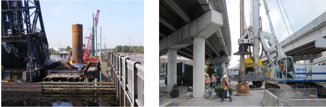
Figure 3.6 Drilled Shafts for Bridge Foundations where Small Footprint is desirable.
