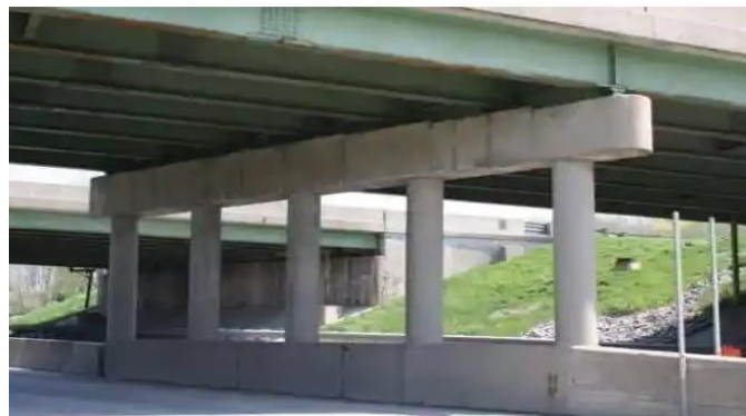
Figure 2.11 Pile Bent Pier
