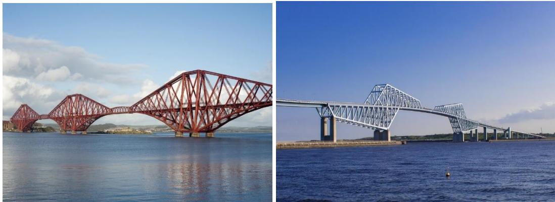
Forth Bridge (UK)
