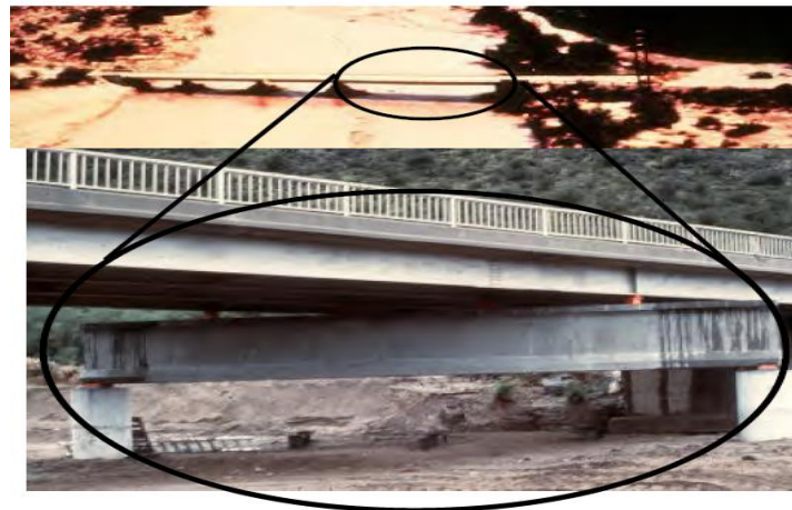
Figure 3.9 Drilled Shafts Installed for Deep Scour Problem
