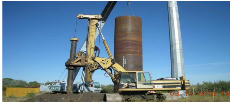
Figure 3.10 Drilled Shafts with Low Headroom
