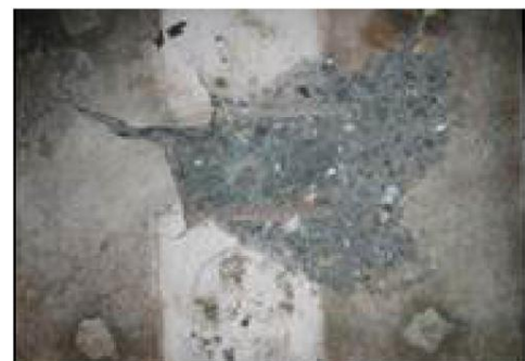
(b) concrete surface
