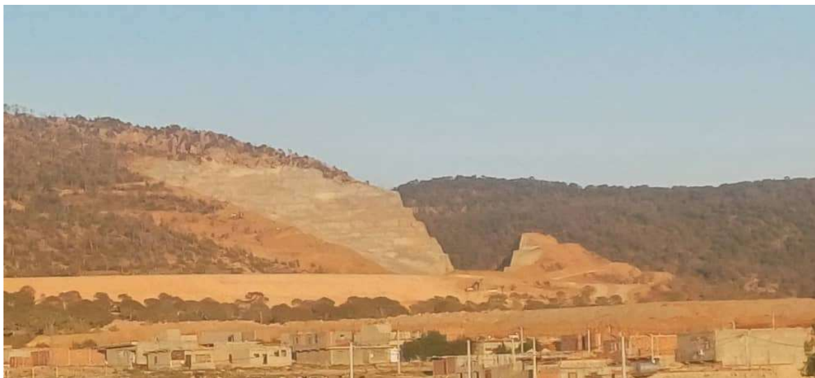
Figure 13 : the railway embankment and the trench excavation site.
