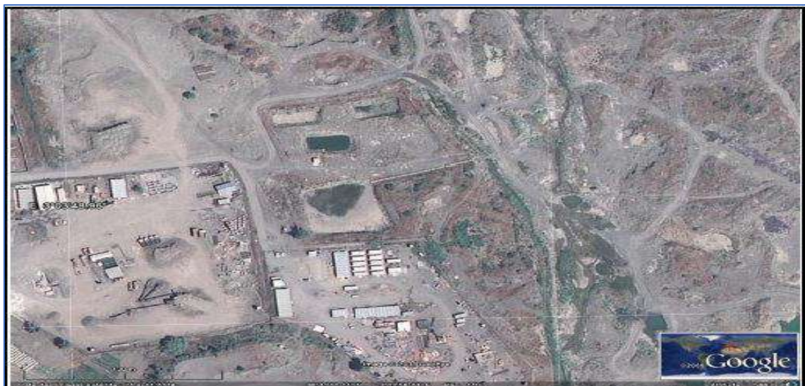
Figure 46: Bassin infiltration (photo Google Earth). (in Djerad Hassiba.2015)
