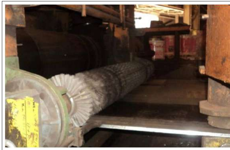
FIGURE 2.5 – Nettoyage du tube [12]
